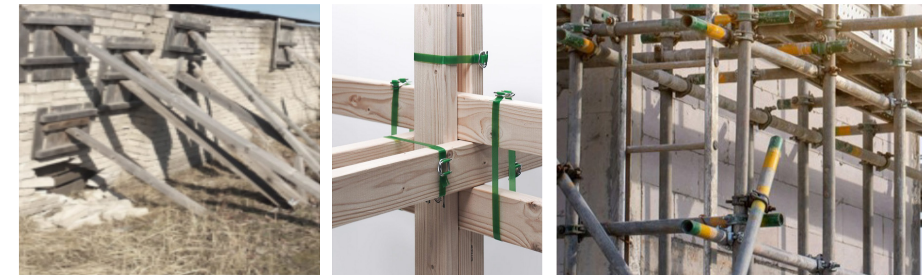
Grid system made of primary beams and secondary battens. The grid size and span can vary depending on the roof elements available. wood, articulations, scaffolding structure...
