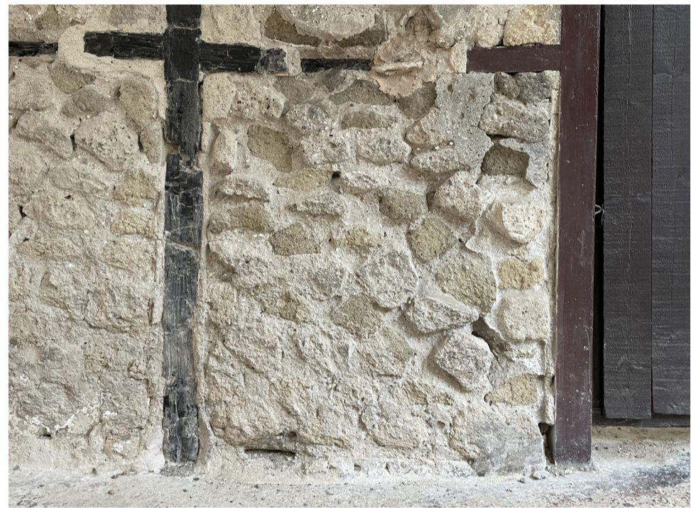
Wooden infill structure at Archeological site of Ercolano, Italy, dated 79 AD. Note the original conserved black wooden part and the new brownish.
