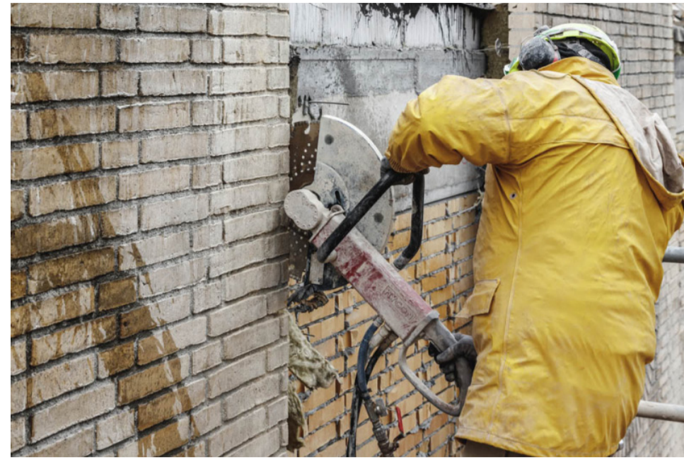
Acquisition of existing brick wall with aim to reuse it in new project. Lendager Studio - Resource rows, 2017
