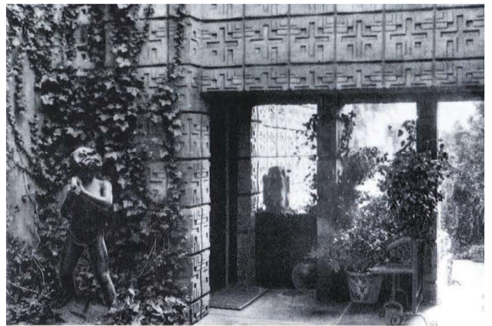
Frank Lloyd Wright - Textile block system. Started as an "experiment" the system was realised six houses. 1920-s.
