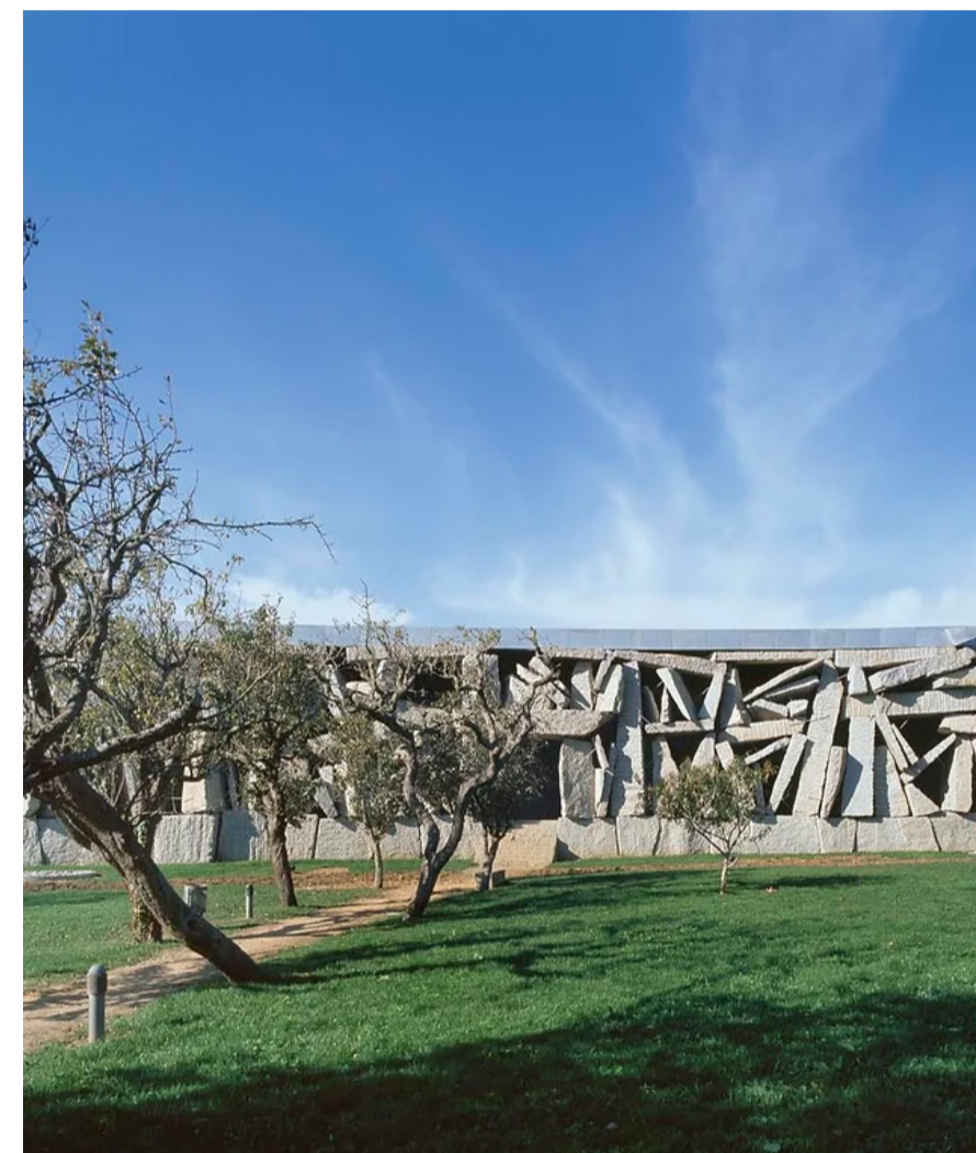
Exterior wall assembly using irregular stone blocks / Ensemble Studio
