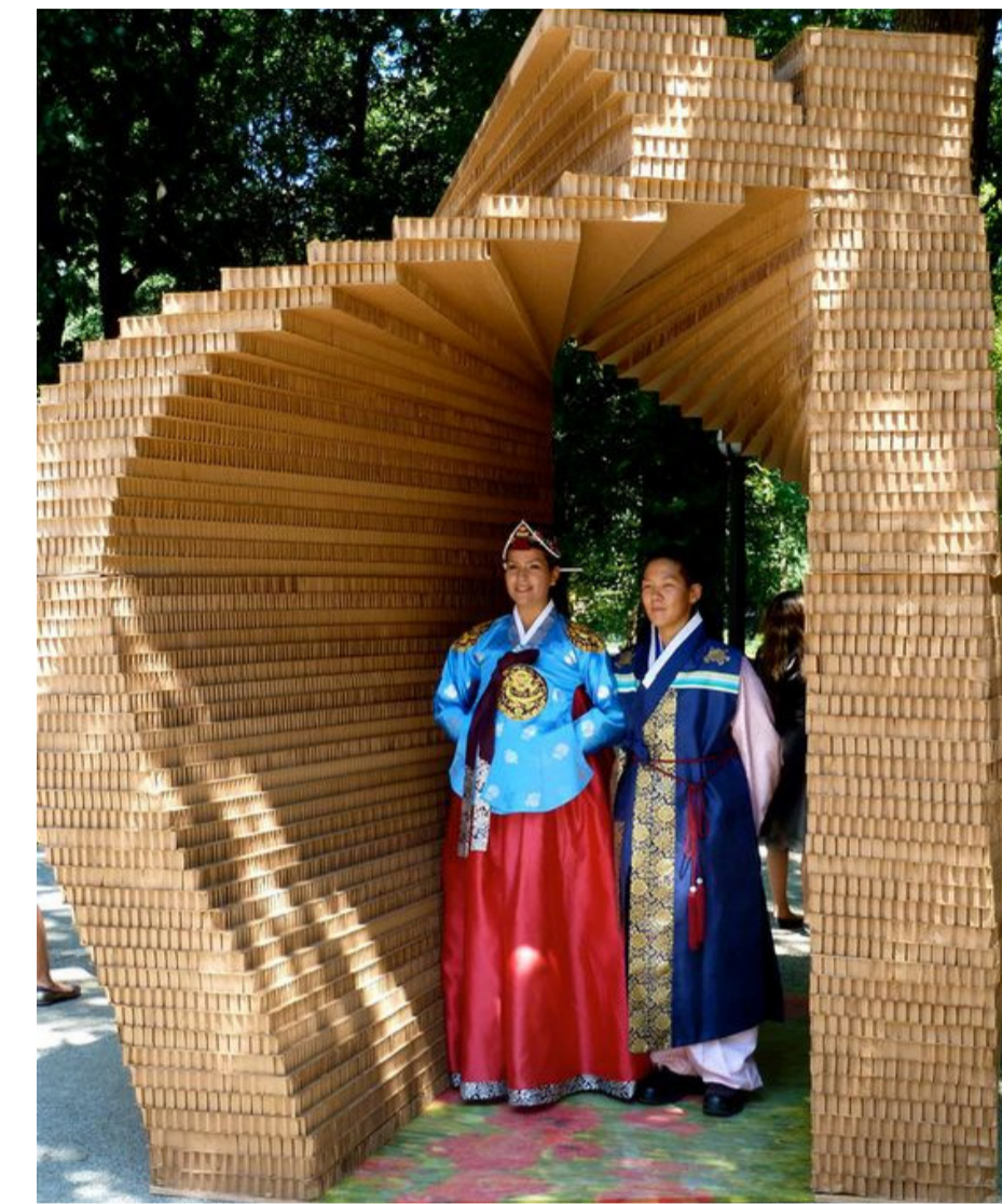
KISS Pop-Up Chapel constructed from stacks of card board panels / Z-A Studio
