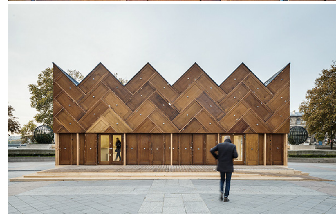
'Circular Pavilion' constructed from re-purposed doors / Encore Heureux
