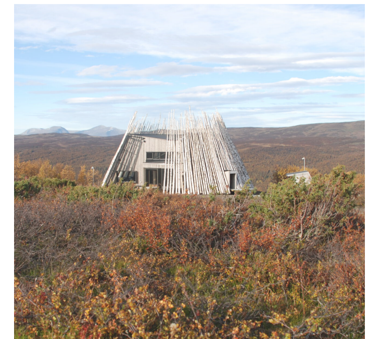
Use of raw wood branch cladding creates a contrast between alignment and mis-alignment / Murman Arkitekter
