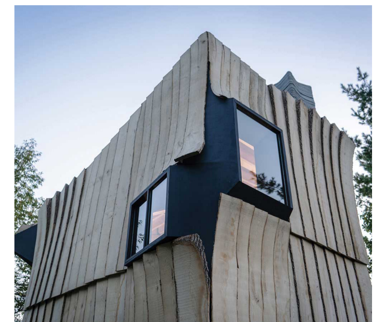
Ashlen Cabin clad by sliced raw wood brings in irregularity and variation to the rigid form / HANNAH
