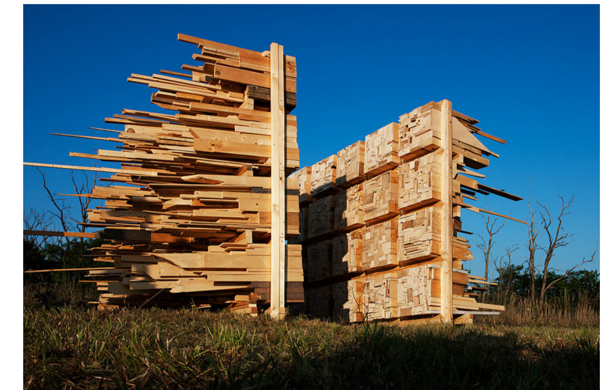
Pavilion constructed from scrap wood with intentional alignment to create differentiated texture on both sides / Hello Wood Architecture Camp
