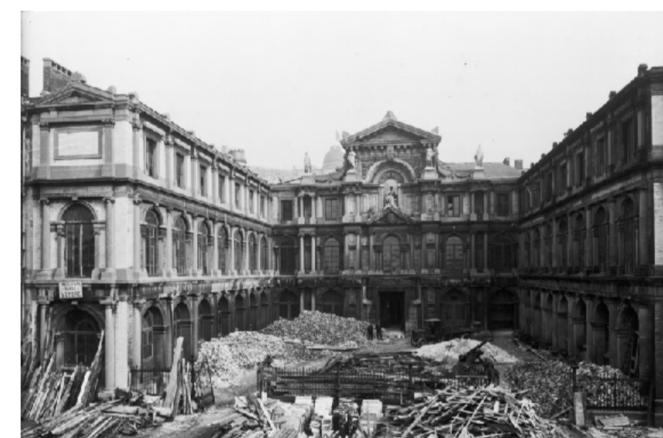
Palais Granvelle Brussels demolition 1931, demolition site as material market
